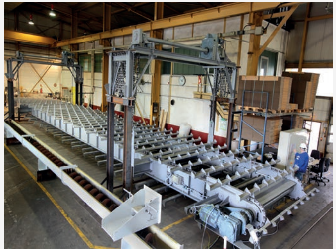
Feedex™ overhead reclaimer
